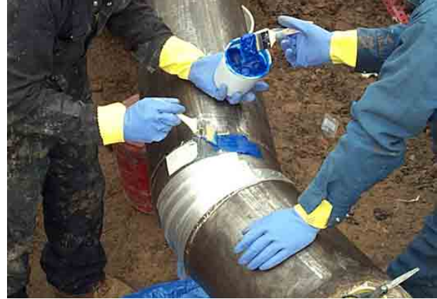
The Anchor Pad, PermaPutty Filler and PermaGrip Adhesive are then applied per Installation Procedure.
