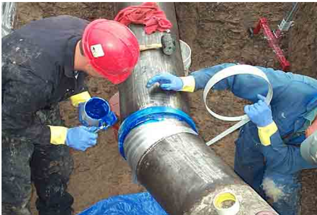
The protective backing is removed from the Anchor Pad. The sleeve is then attached to the Anchor Pad and applied to the pipe per standard installation procedure.
