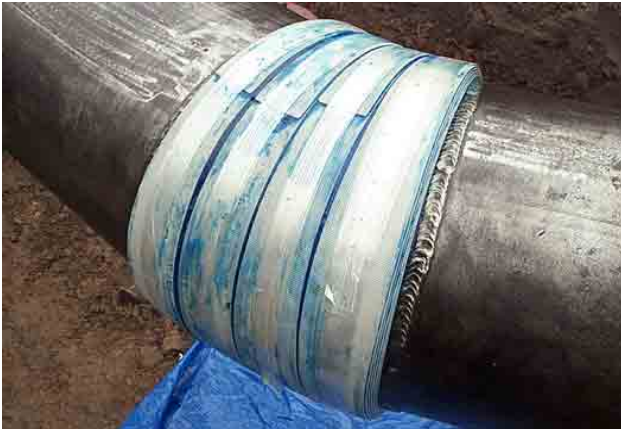
Using a clean rag, wipe the excess adhesive from the bend repair sleeves. A rag with a small amount of solvent may be used to assist cleanup. If repairing corrosion near the girth weld, apply a PermaWrap sleeve butted to the other side of the girth weld, using the traditional girth weld repair procedure.
