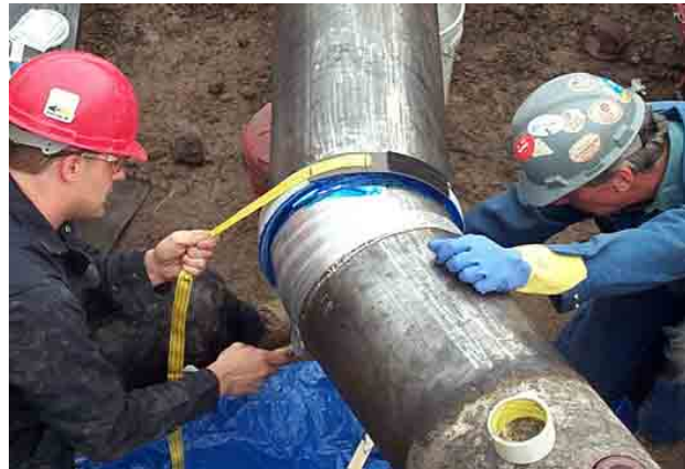
Using the narrow Velcro strips supplied in the kit, the torque bar strap is attached to the sleeve and tightened per installation procedure. Be careful not to over torque and pull the sleeve from the Anchor Pad.
