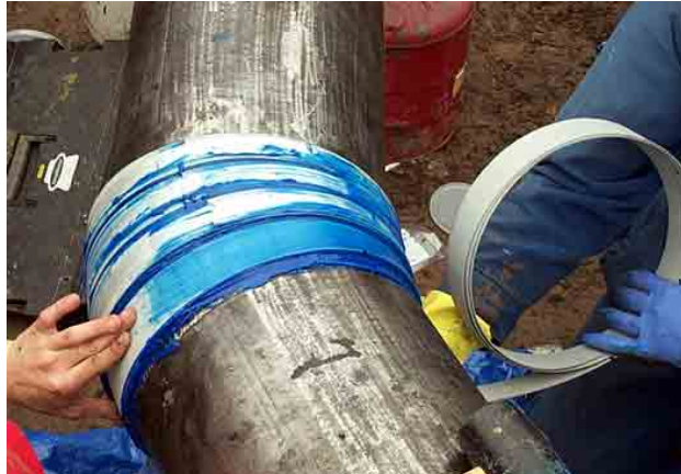
Upon completion of the last numbered PermaWrap sleeve, remove all the excess PermaPutty filler and PermaGrip adhesive.
